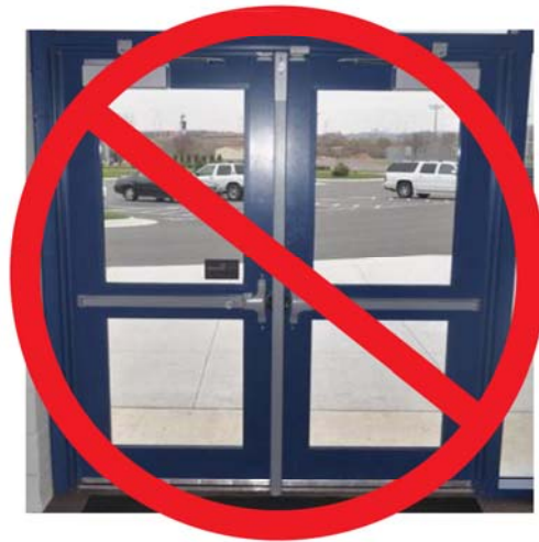
Traditional removable mullions are unsightly and do not fix air and water infiltration.
